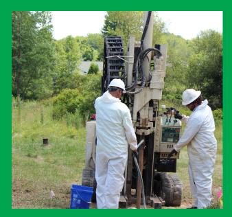
Cascade Remediation Services crews provide calculated injections to remediate soil and groundwater contamination.
