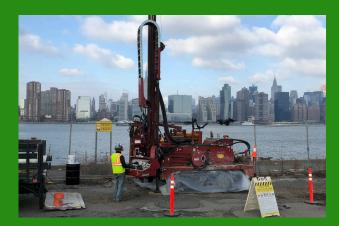
ADT provides geotechnical and environmental drilling services to the greater New York City area.
